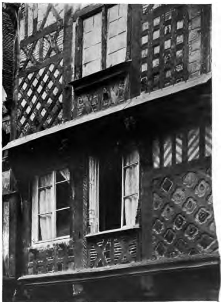
BEAUVAIS. HOUSE FRONT, c. 1550. TIMBER WORK SET WITH COLOURED POTTERY
